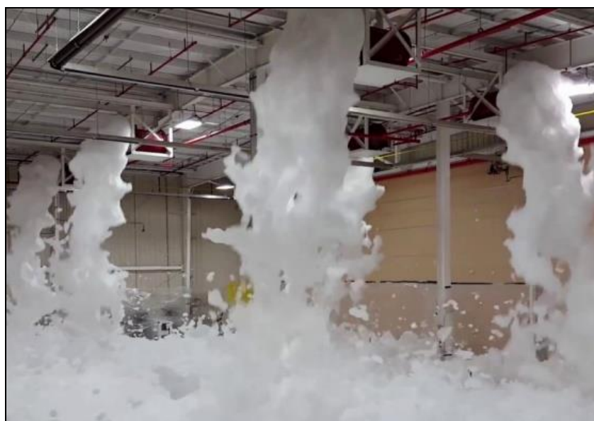
High expansion foam system operation in a warehouse
