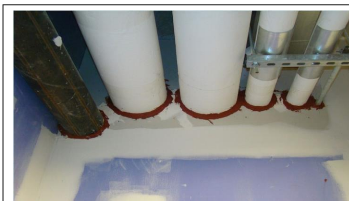
Through penetration barriers around pipe penetrations
