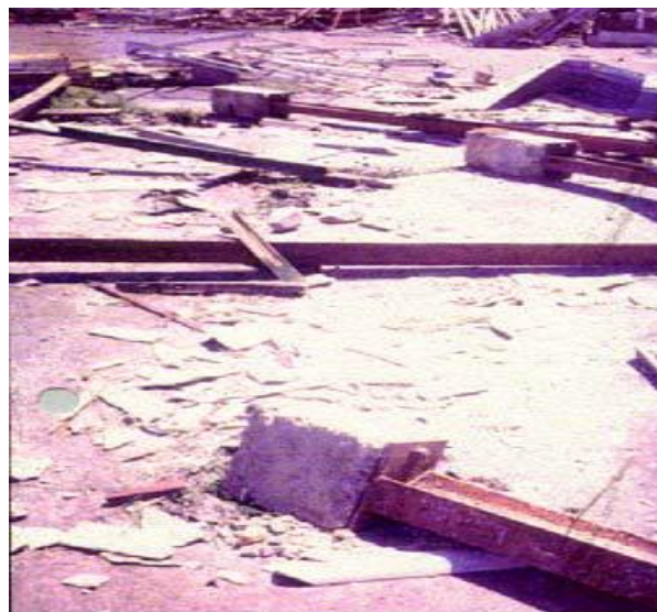
Foundation of a steel framed light weight structure completely pulled out of ground
