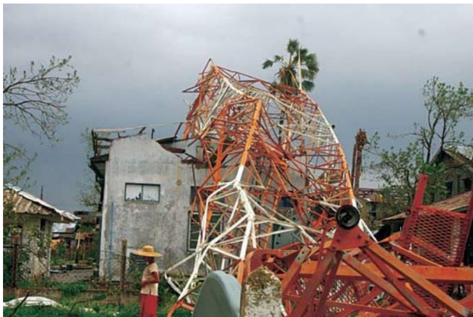
Figure 7: Cyclonic wind disrupting communication towers ( Source: SoP, RSMC Delhi )
