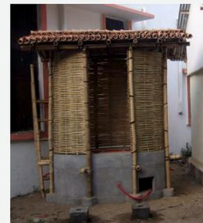
*EcoSan toilet constructed using bamboo for flood affected areas*
