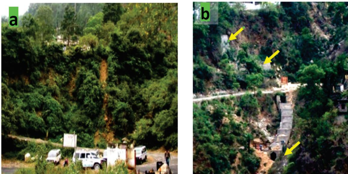
**Figure 1** a) Landslide at Karnaprayag before mitigation; b) after structural mitigation at the initiative of District & Tehsil/Block Disaster Management Committee through coordinated efforts of the stakeholders (DMMC, 2003 & Uniyal, 2004 & 2016)
