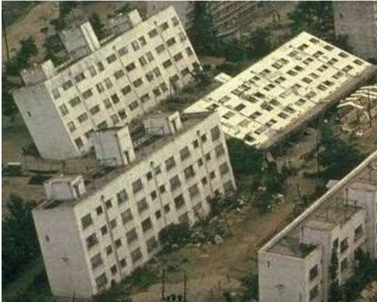
Soil liquefaction in 1964 Niigata Earthquake
