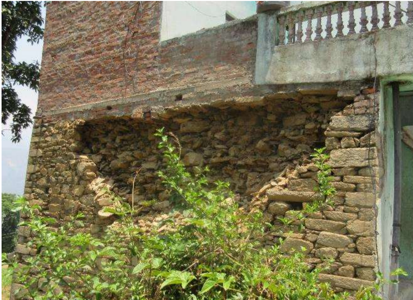
Delamination of stone wall
