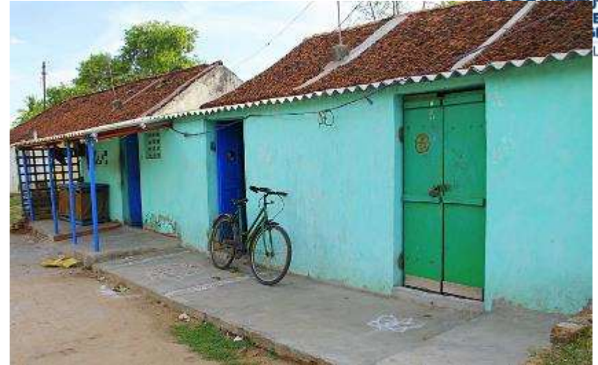
Burnt Brick walls with country tiles gabled roof- West Bengal
