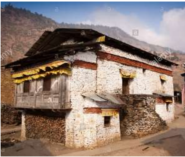
Stone rubble masonry walls with CGI sheets gabled roof- Jammu & Kashmir
