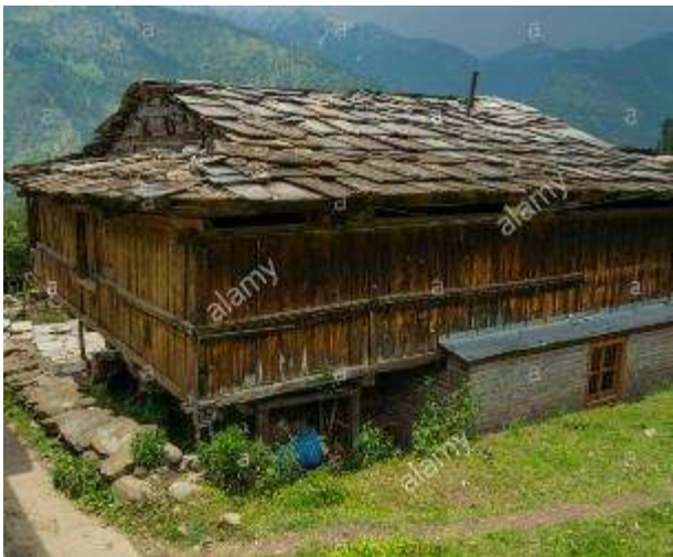
Timber walls with slate stone hipped roof- Himachal Pradesh
