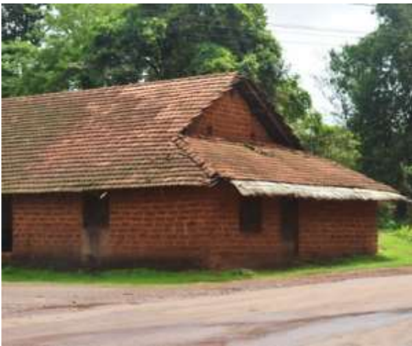
Ashlar Stone Walls with Mangalore tiles hipped roof- Goa
