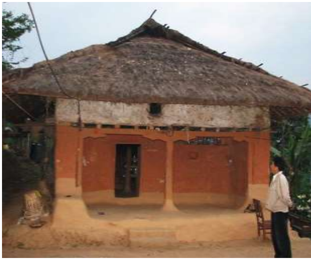
Adobe walls with thatch hipped roof - Sikkim
