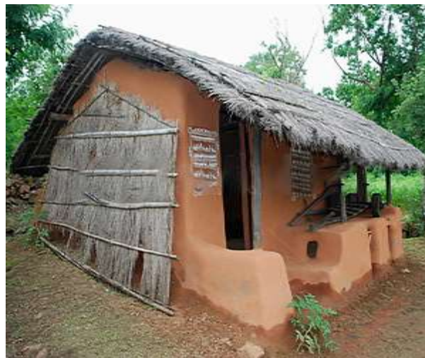
Cob walls with thatch gabled roof - Madhya Pradesh
