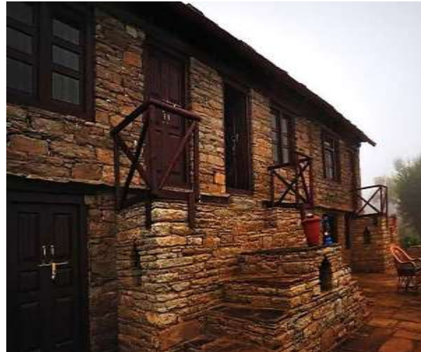
Stone rubble masonry walls with mangalore tiles gabled roof- Uttarakhand
