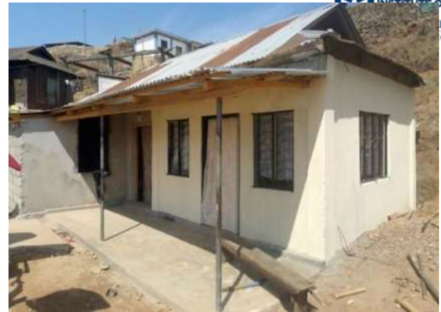
Burnt Brick walls with CGI sheets gabled roof- Meghalaya
