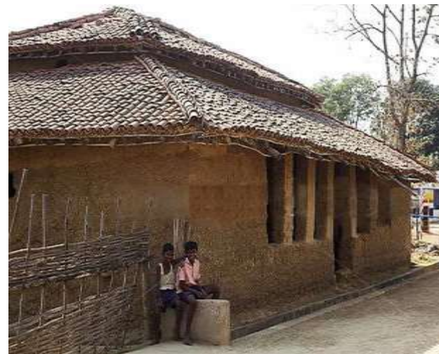
Cob walls with tiled hipped roof - Chhattisgarh
