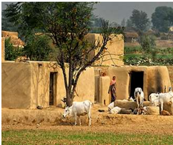
Cob walls with timber and mud flat roof - Haryana
