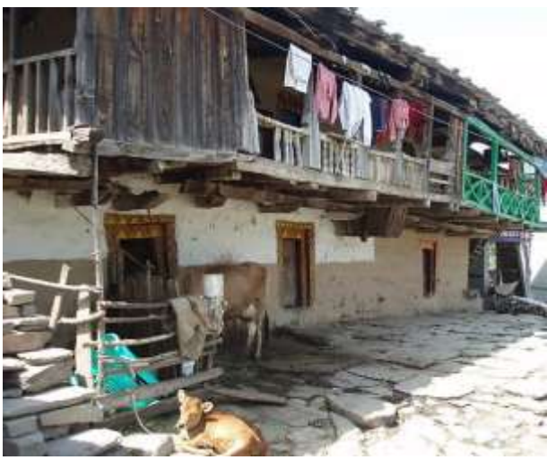
Timber walls with timber gabled roof- Uttarakhand
