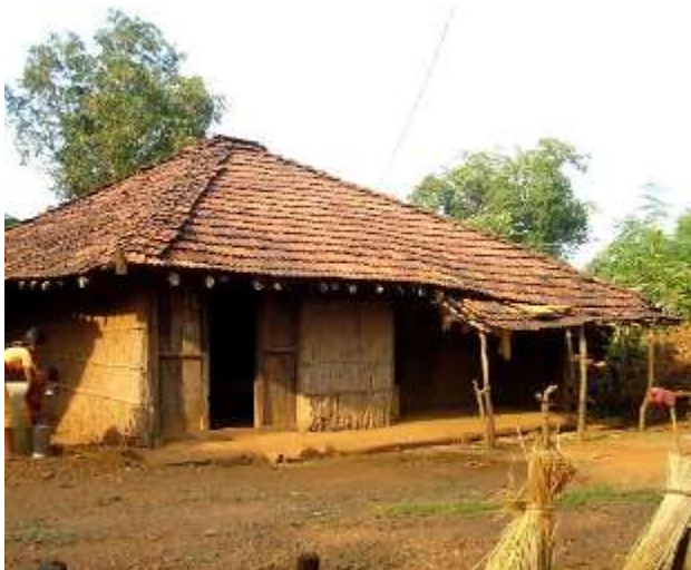
Wattle and daub walls with Mangalore tiles hipped roof - Maharashtra
