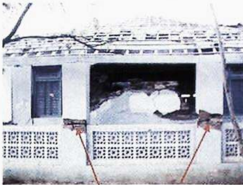
Masonry column cracking
