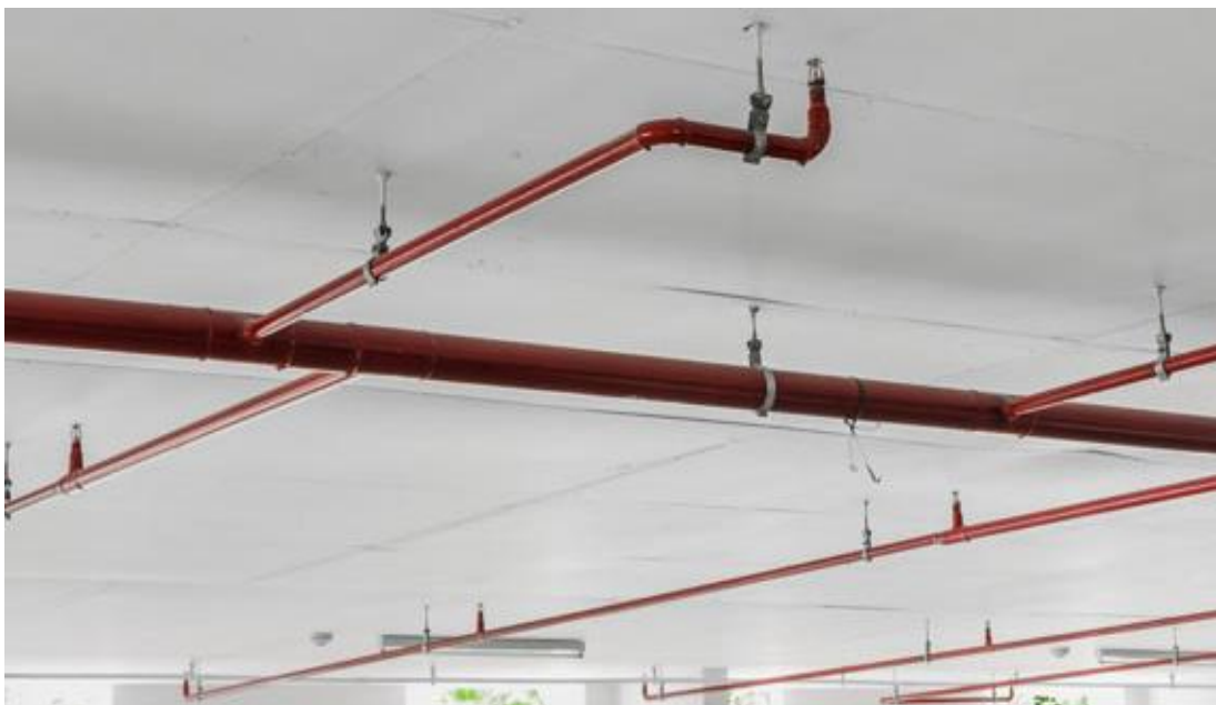
Automatic Sprinkler System
