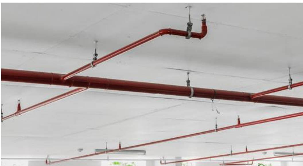
Automatic Sprinkler System
