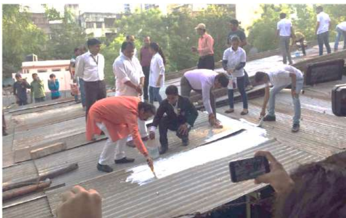
Figure 20: Ahmedabad mayor initiating cool-roof
